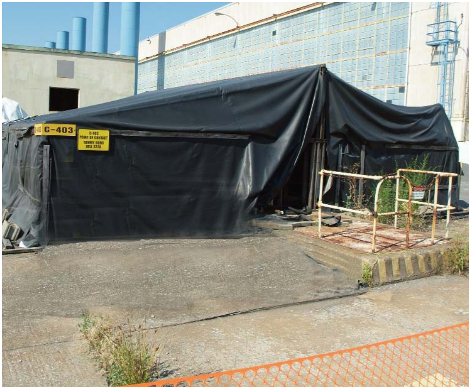
The C-403 Neutralization Pit is one of three inactive facilities with soil contamination included in the Soils Operable Unit.
