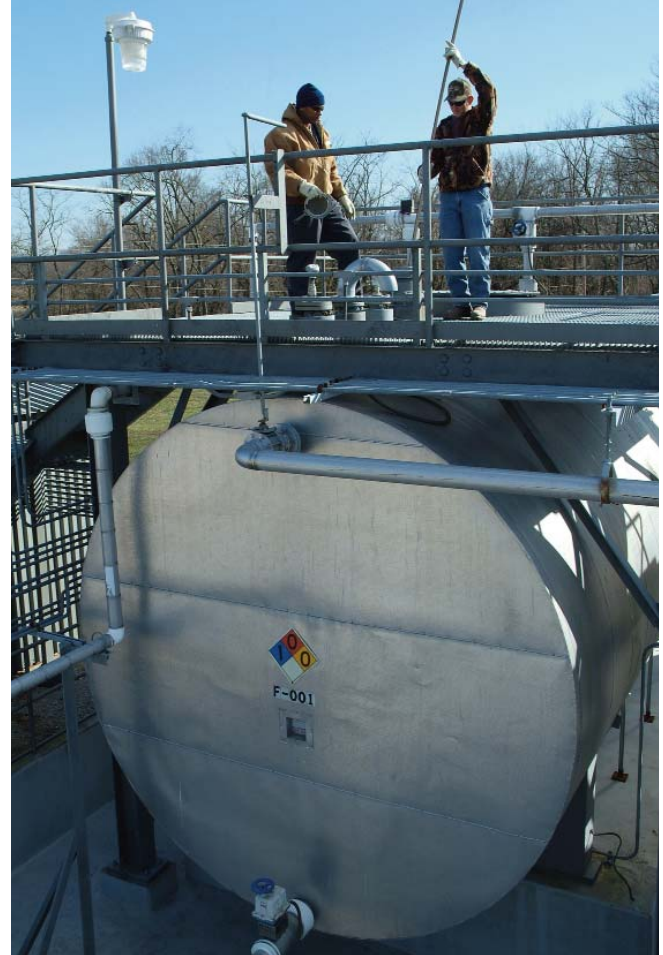
The water level in one of the landfill's 31,000-gallon leachate storage tanks is measured.
