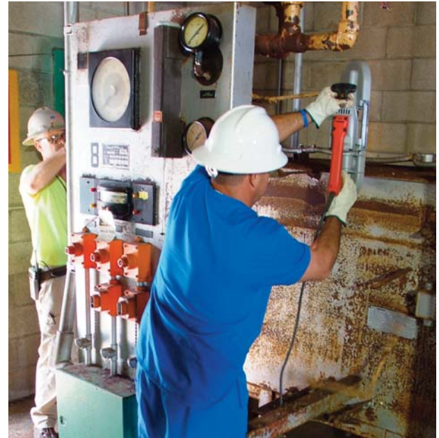
Workers remove pipes leading to process equipment located inside C-342.
